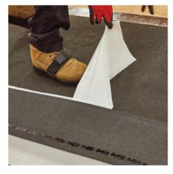
Peel and stick design eliminates the need to cut and nail starter strips
