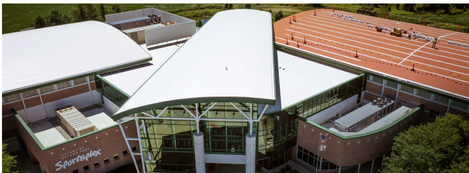
Two coats of GAF High Solids Silicone Roof Coating System over a base coat of GAF Multi-Purpose Primer preserved the integrity of the acoustic Orlando Sports Park roof.
