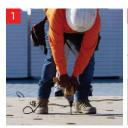
Attach insulation or cover boards to deck using Drill-Tec™ RhinoBond® Plates and Fasteners.
