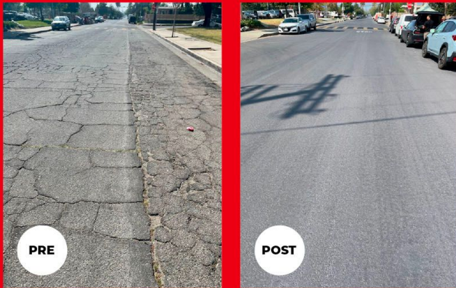
Figure 2: Filmore Street Pre-/Post-Installation
